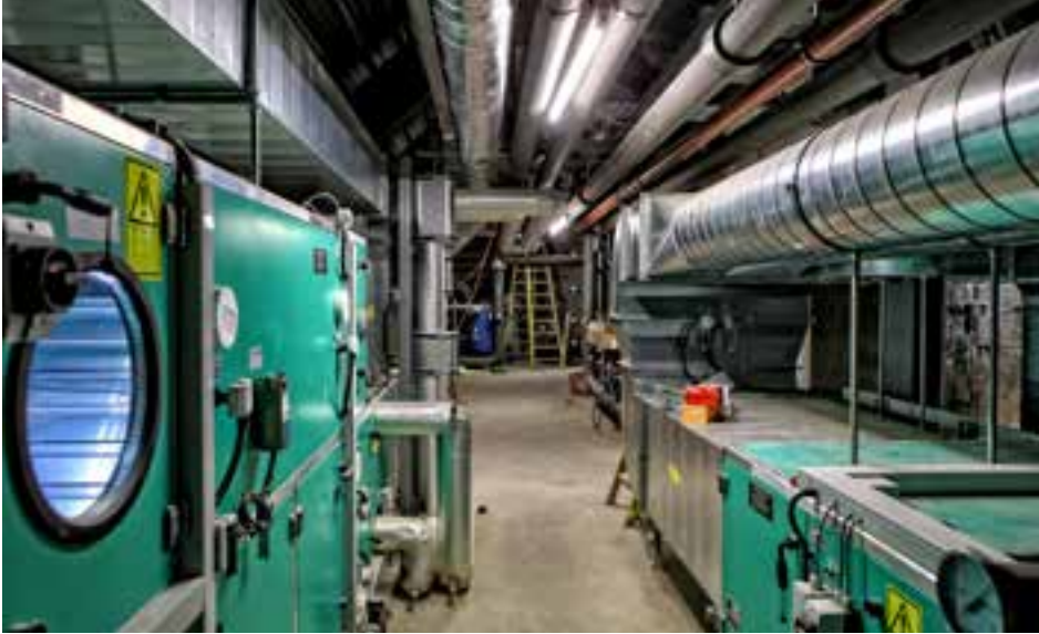
The technology floor (6 th floor, attic), where all the technical installations of the building are located, includes a photovoltaic system (horizontal- and bevels). The produced electricity is fed directly into the grid of Sika.
