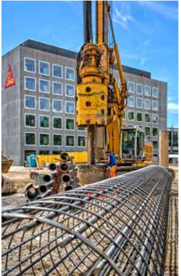
Due to the ground conditions and the building's design, the foundations required several different types and sizes of piles.
